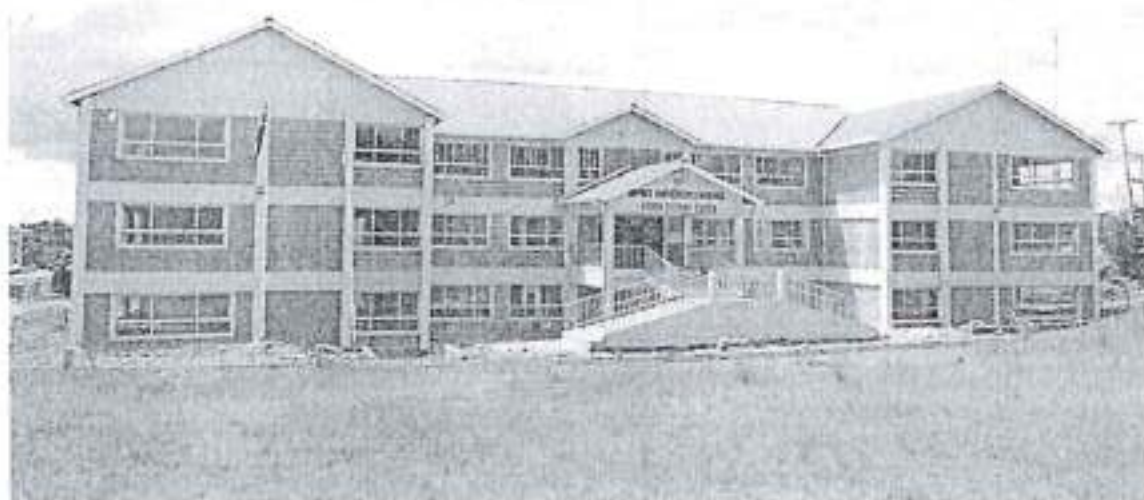
Picture 2: BUC Green Tuition Block- Inside square (99% completion)
